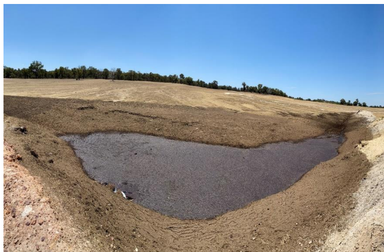
Figure 2: Looking upslope at a silt trap that has captured sheep faeces from a storm event.
